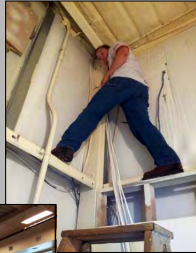
Chris Roertgen installing CCTV cables at Lighthouse Mission.
