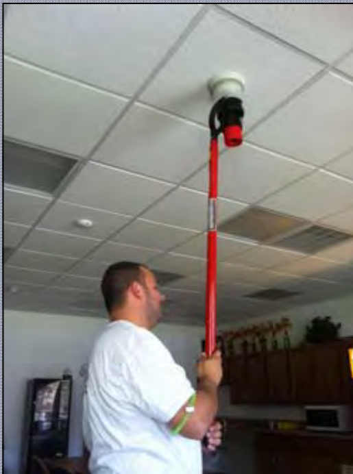
Below, Briscoe tech Jeff Kempf tests a smoke detector
