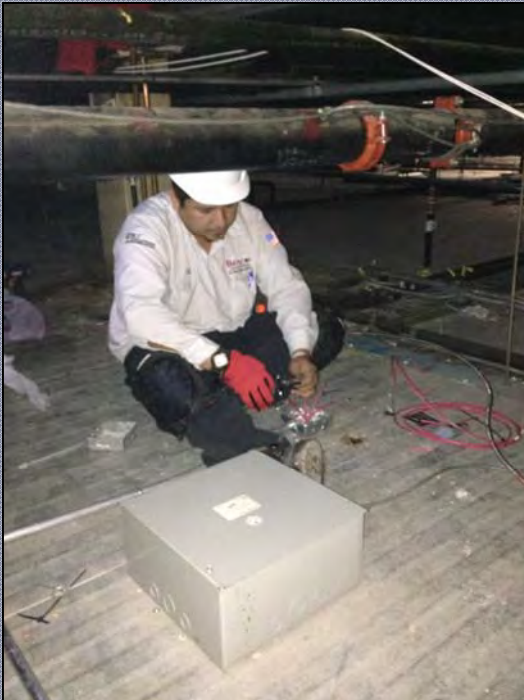
Below, Briscoe tech Steve Vargas adds fire alarm devices to a system
