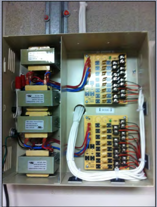
Above, field wiring of CCTV power supply is neat and orderly
