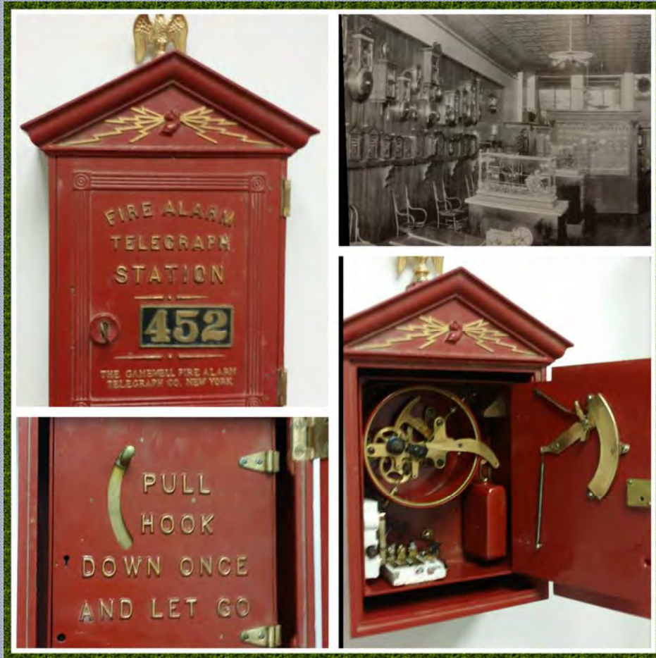
NYC Fully Functional Fire Alarm Telegraph Station circa 1869. (Made by Gamewell when they were in NYC) Gamewell Show Room in NYC pictured as well."
